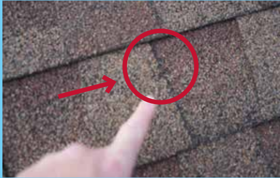
Actual hail damage in Legacy Oaks—damage not visible from the ground. We offer drone inspections for safety.
