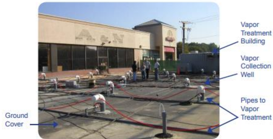
ERH system cleans up contaminated soil and groundwater.
